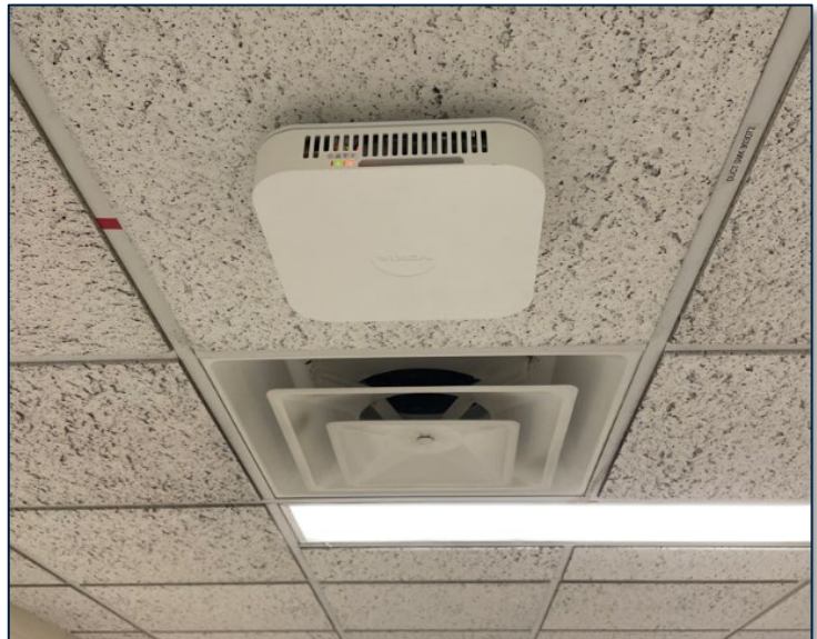
Figure 6 Nokia MBO and antenna mounted on the roof of Terminal 1
